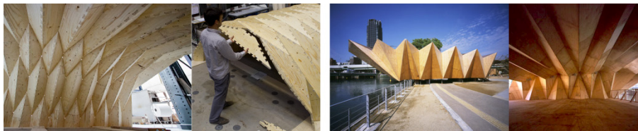
Fig. 2. Interlocking Folded Plate Structure (left) and The Temporary Pavilion (right)
