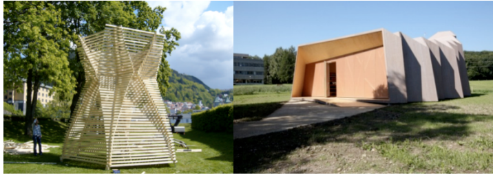
Fig. 2 Example of modulated pilling-up: BWIF Sculptures, Bergen, Norway Fig. 3 Example of tessellation: Saint Loup chapel, Switzerland
