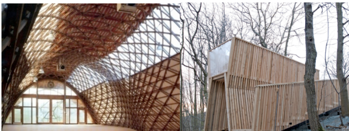
Fig. 4 Example of a mesh: Weald & Dowland museum, Chichester England Fig. 5 Example of Armature: Observation platform, Trondheim, Norway
