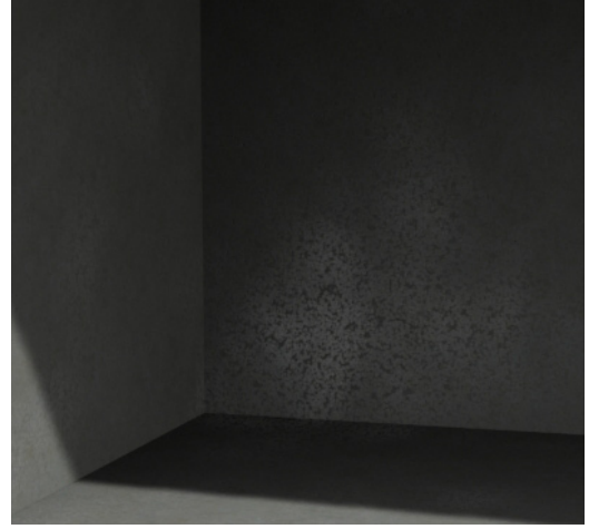
Figure 69: efflorescence, detail
