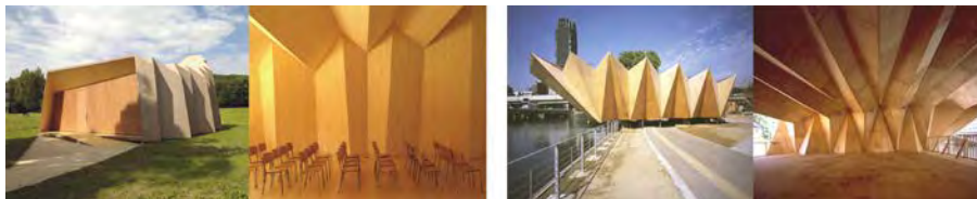
Figure 1. The Chapel of St Loup (left) and The Temporary Pavilion (right).
