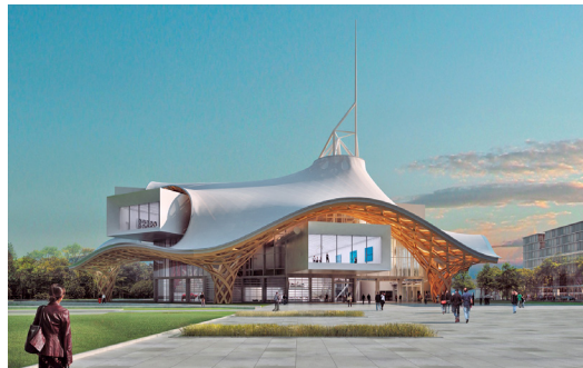
Figure 3 (left) Centre Pompidou, Shigeru Ban, Metz, France
