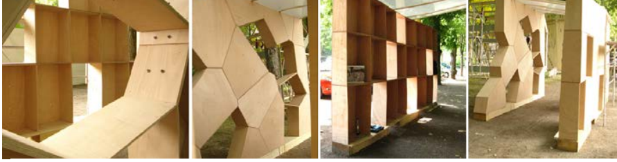
Figure 8. Finished wall prototypes. A, Grid-pattern wall view through a voronoi cell. B, Voronoi-patterned wall. C, Grid-pattern finished wall. D, Finished prototypes.
